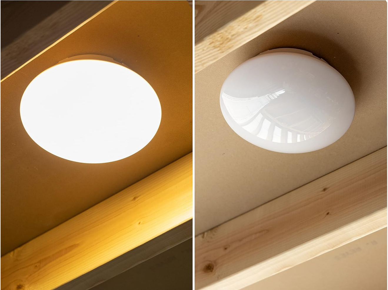
Image 5.2: Demonstration of the 60-minute automatic shut-off timer.
