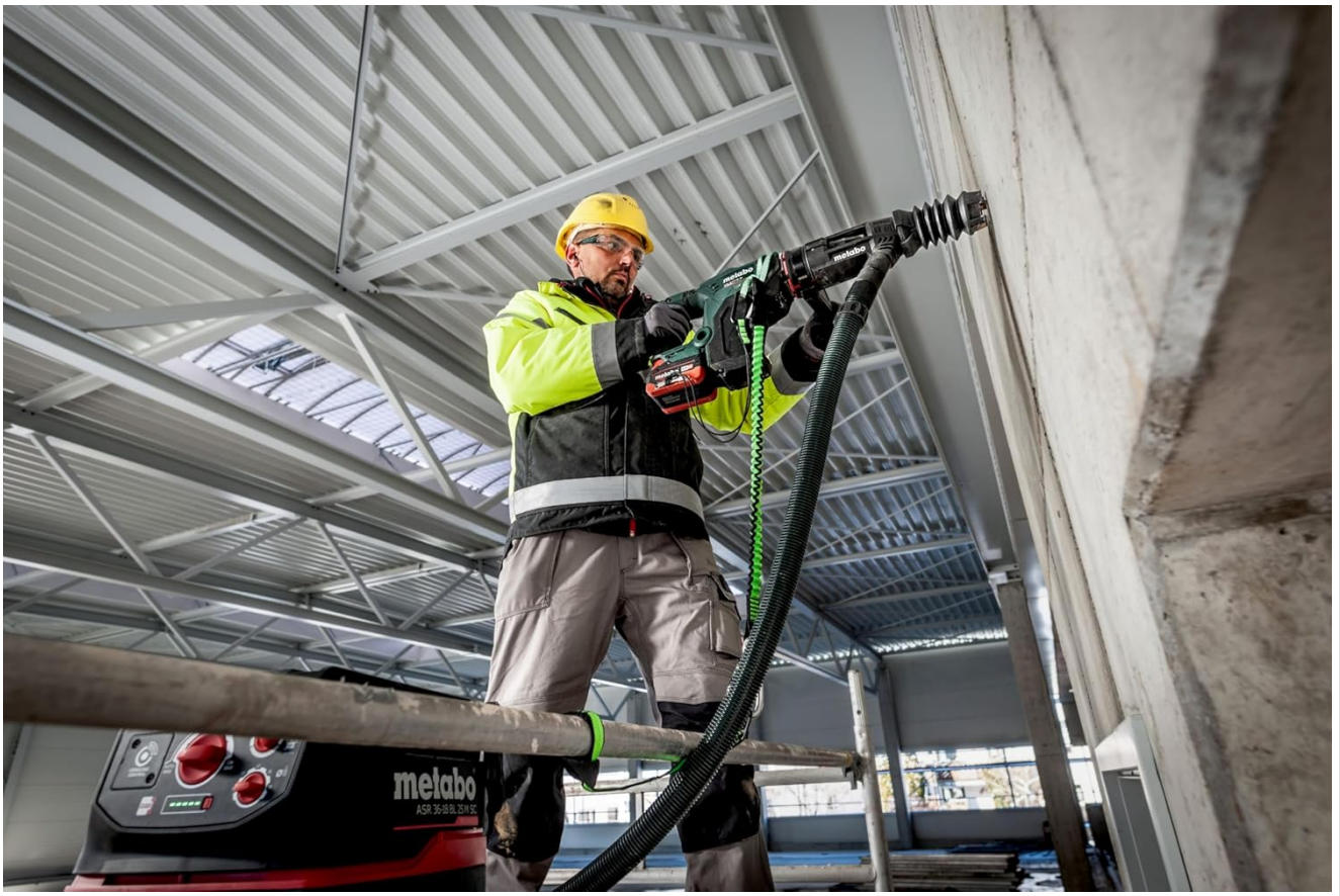
Figure 4.2: An individual performing overhead drilling with the Metabo KHA 18 LTX BL 40, demonstrating the use of the tool in an elevated position, also connected to a dust extraction unit.
