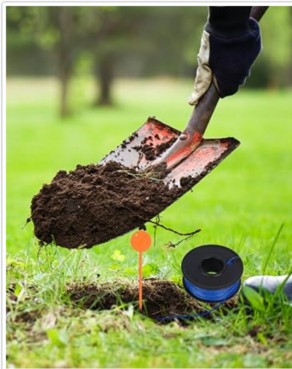
Image: A close-up of a person using a shovel to bury the blue boundary wire in a grassy area, with a white training flag visible nearby.
