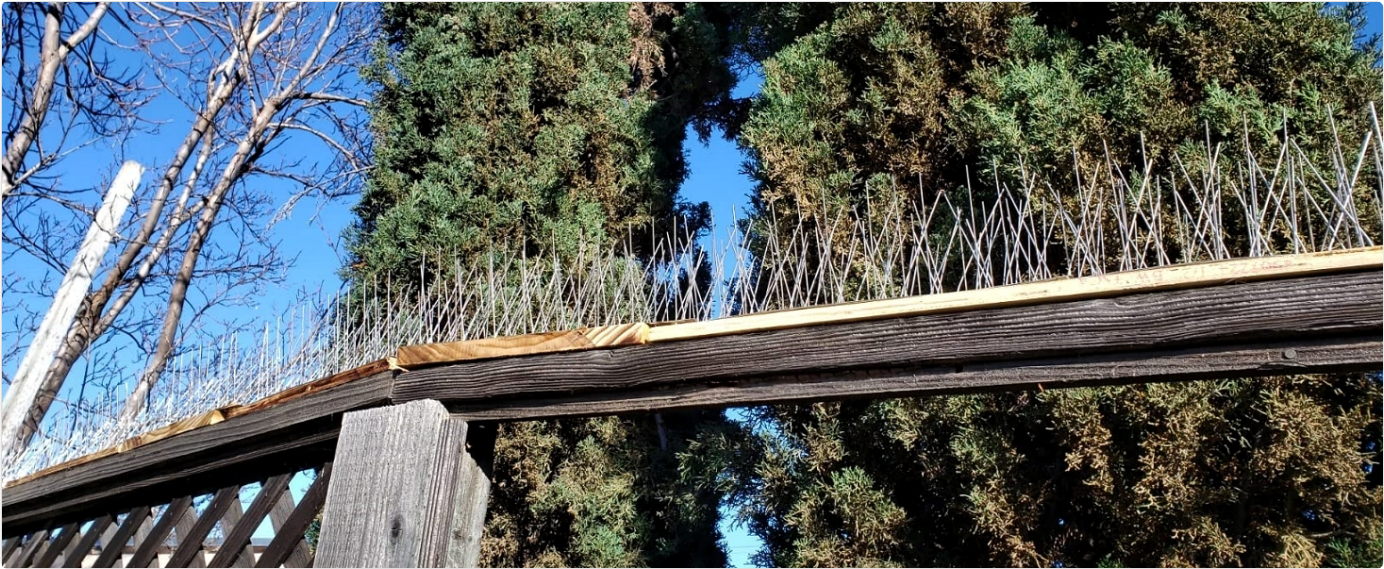
Image: Examples of ineffective spike placement, highlighting the importance of full coverage and proper density.
