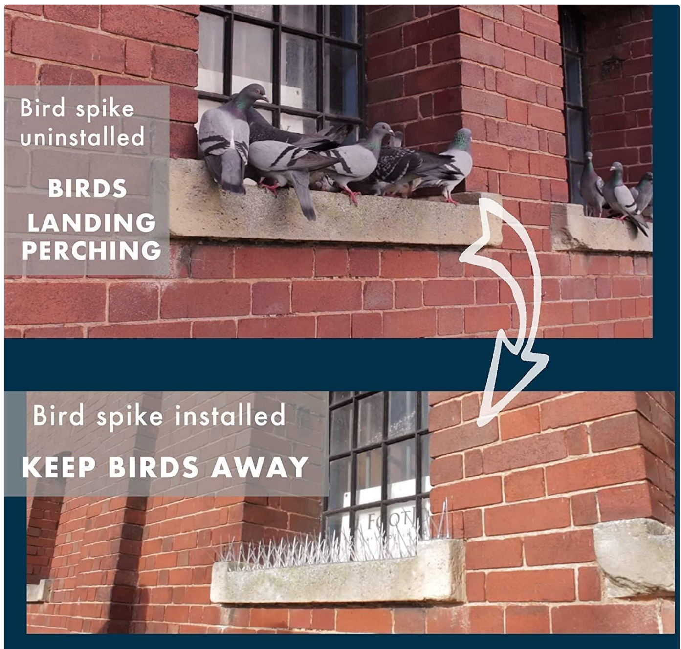
Image: A visual comparison demonstrating the effectiveness of bird spikes before and after installation on a window ledge.
