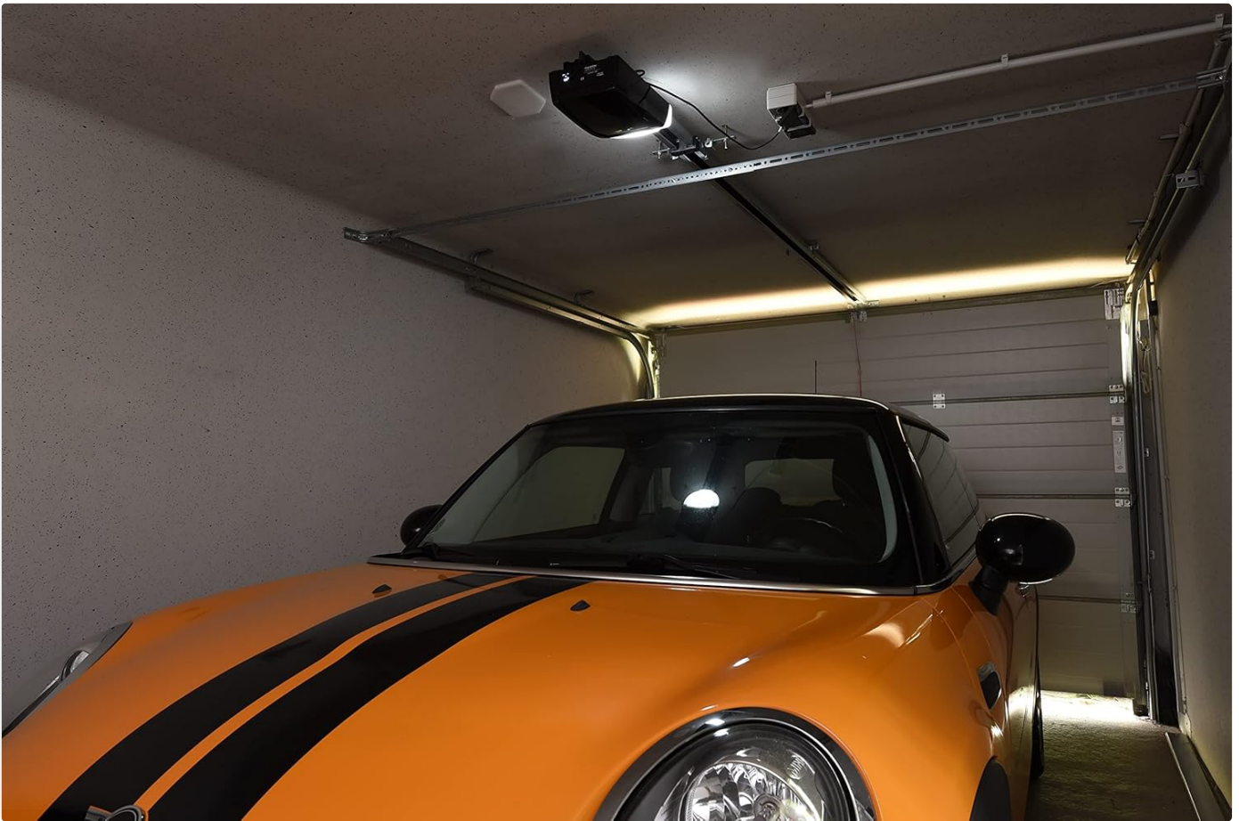
Image: The Marantec garage door operator installed in a garage, illuminating the space with its integrated LED lighting, with a car parked underneath.
