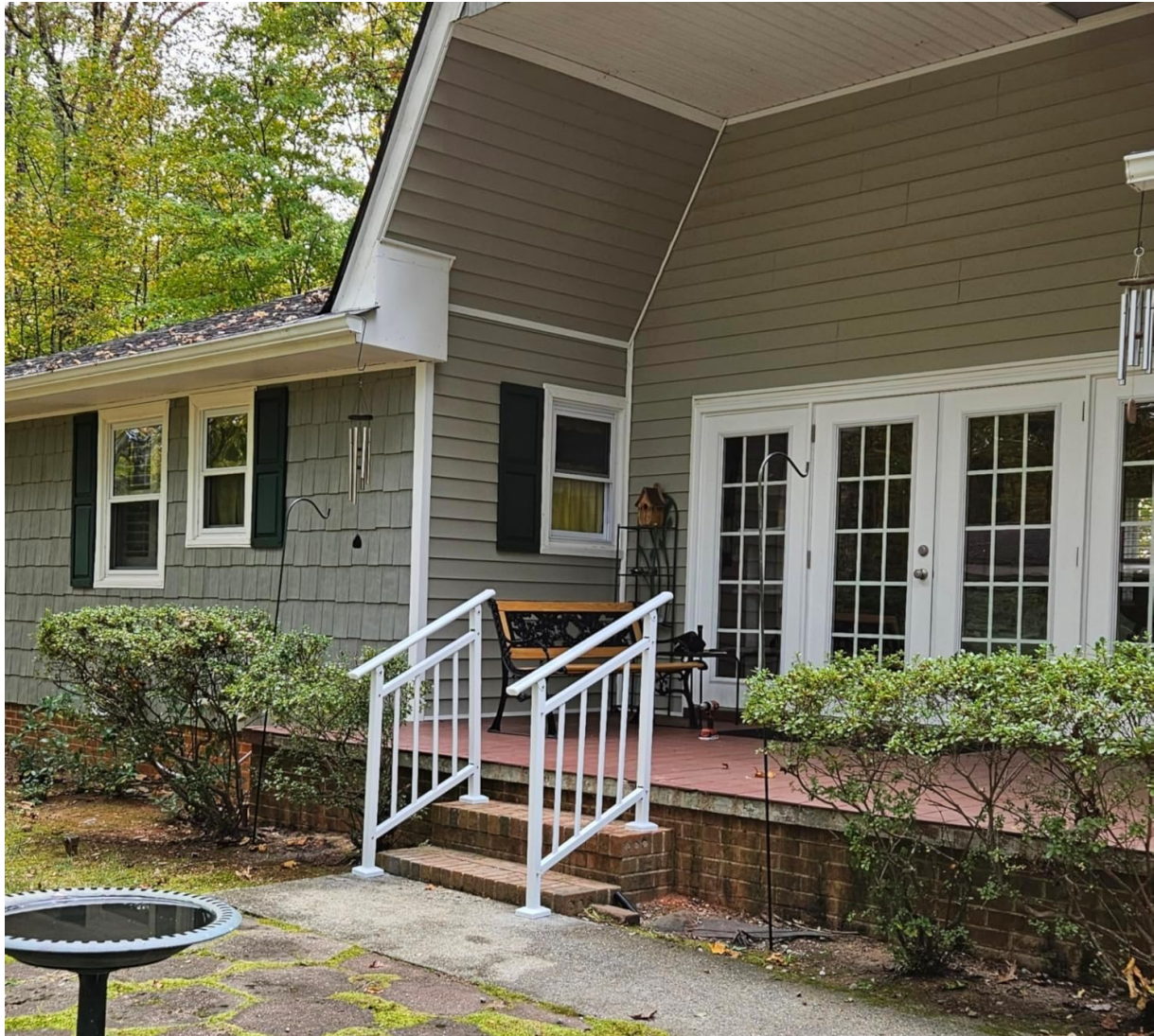
Image 4.5: Example of an installed handrail on a porch.
