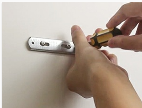
Figure 3: Securing the mounting bracket to the wall.
