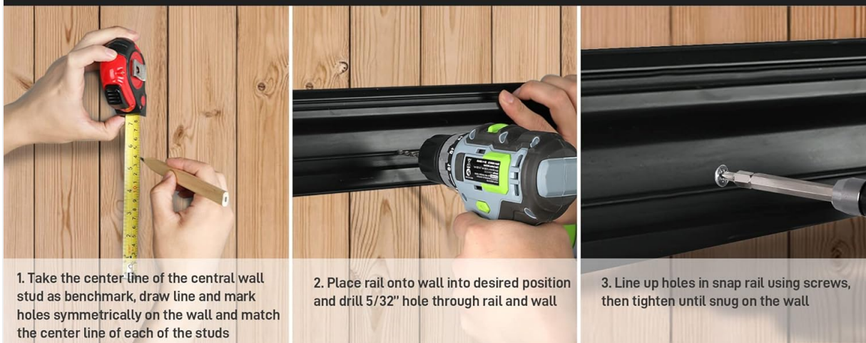
Image 3: Visual guide demonstrating the installation process for the storage rails on both masonry/concrete walls and wood studs, showing drilling and securing steps.
