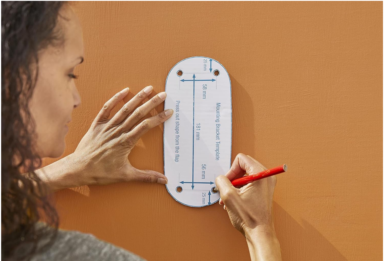
Image: A user marking the wall for bracket installation using the provided template, ensuring accurate placement of drill holes.
