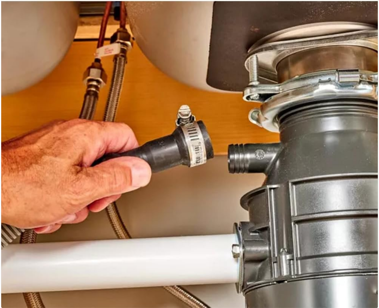
Image 2.2: Demonstrates the easy connection of the hose to a garbage disposal unit.
