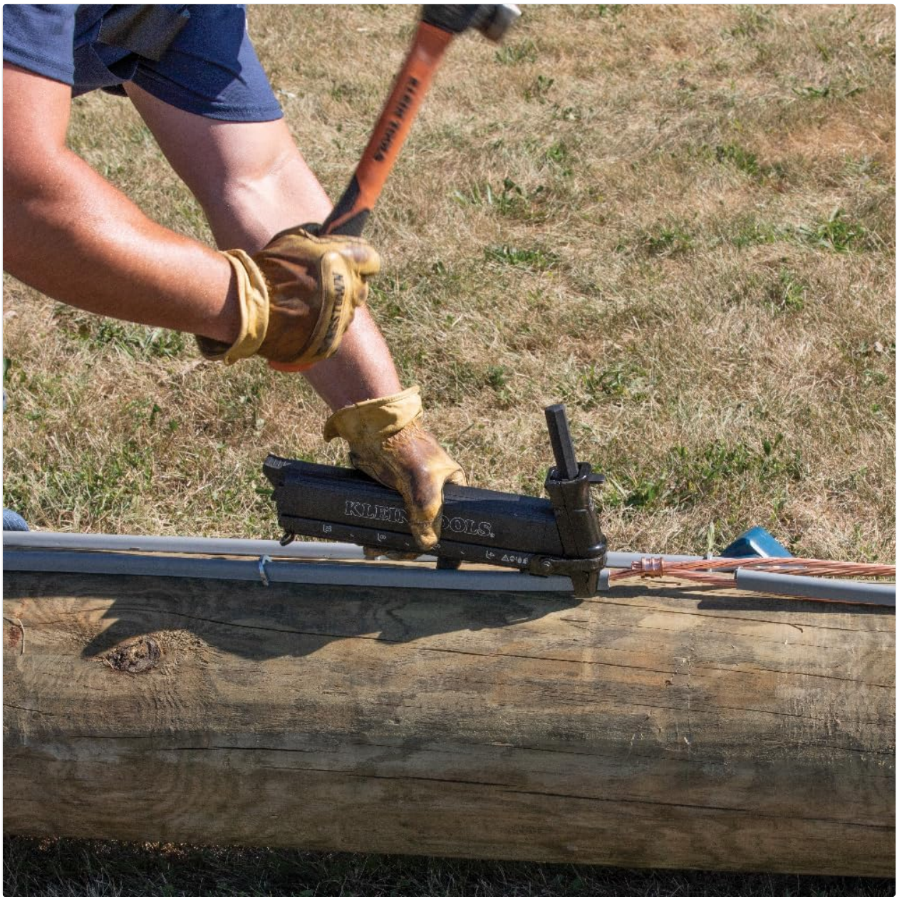
Image 3.2: The staple starter being used to install ground wire, showcasing its application on a utility pole.
