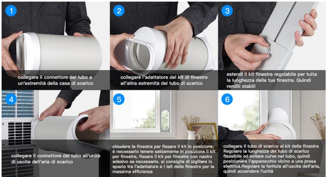
Image 5.1: Detailed steps for exhaust hose and window kit installation.
