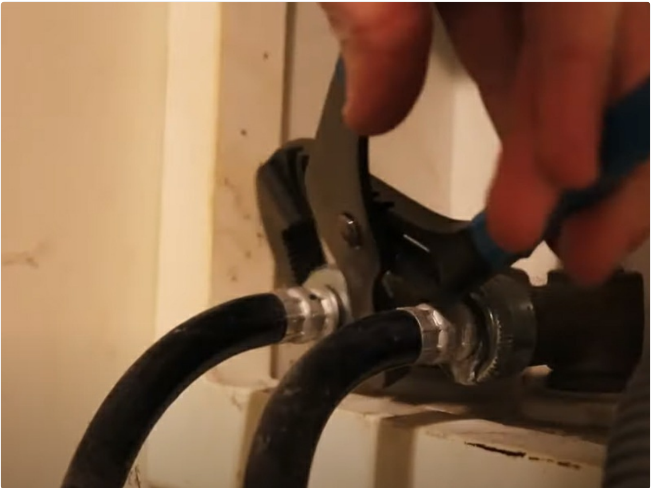
Image: Disconnecting Old Hoses
