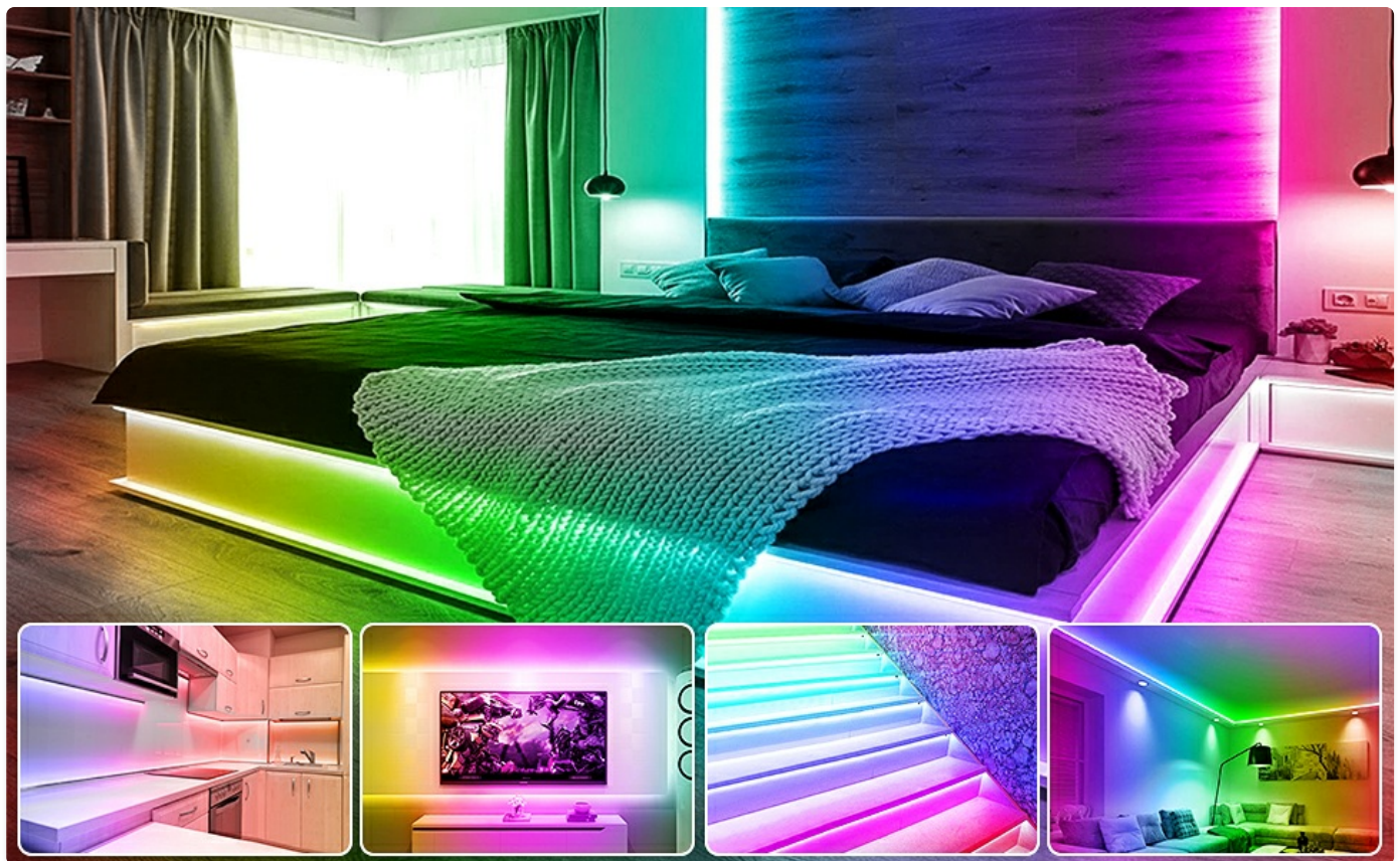
Image 11.2: The LED neon rope light providing colorful ambient lighting in a bedroom.
