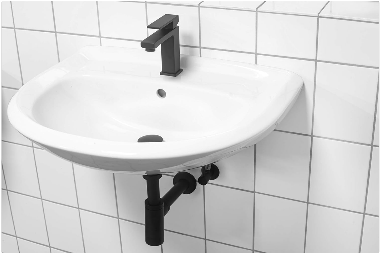
Image: Cornat siphon installed under a basin.
