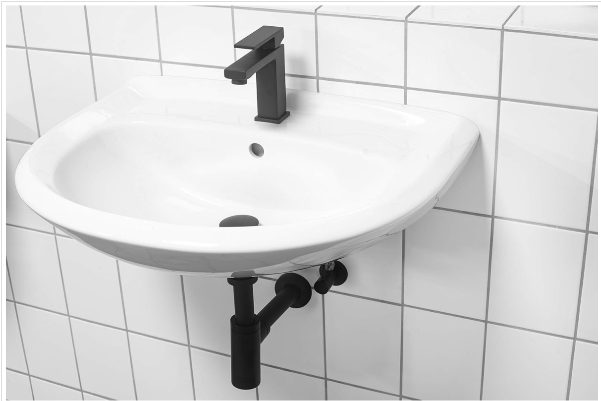
Figure 3: Installed drain valve in a washbasin.
