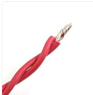
Image 3.2: The stripped ends of two red wires are twisted together, preparing them for insertion into a wire connector.
