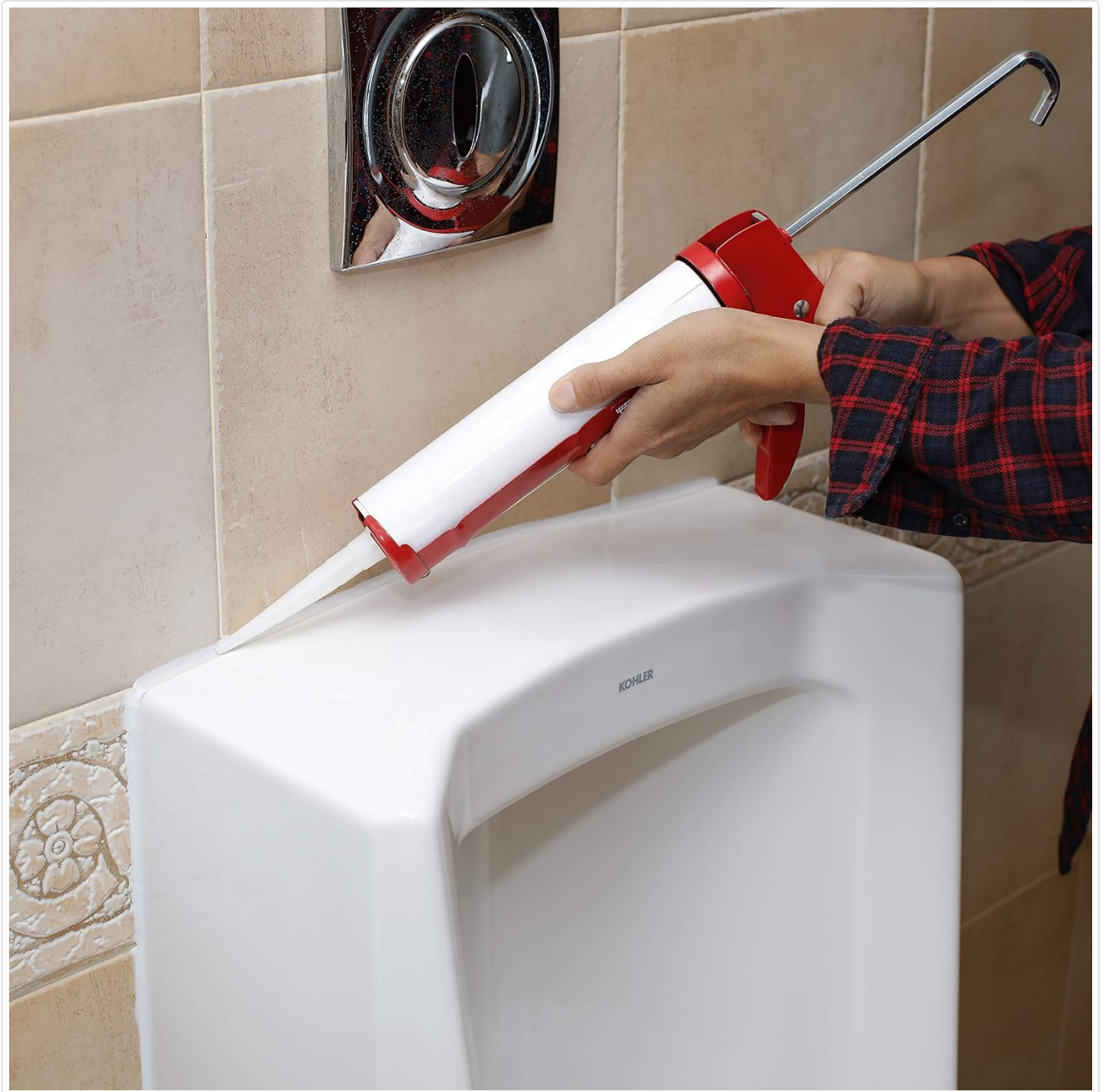
Image: A person using the Hyper Tough 9-Inch Dripless Caulk Gun to apply caulk along a seam, demonstrating proper angle and technique.
