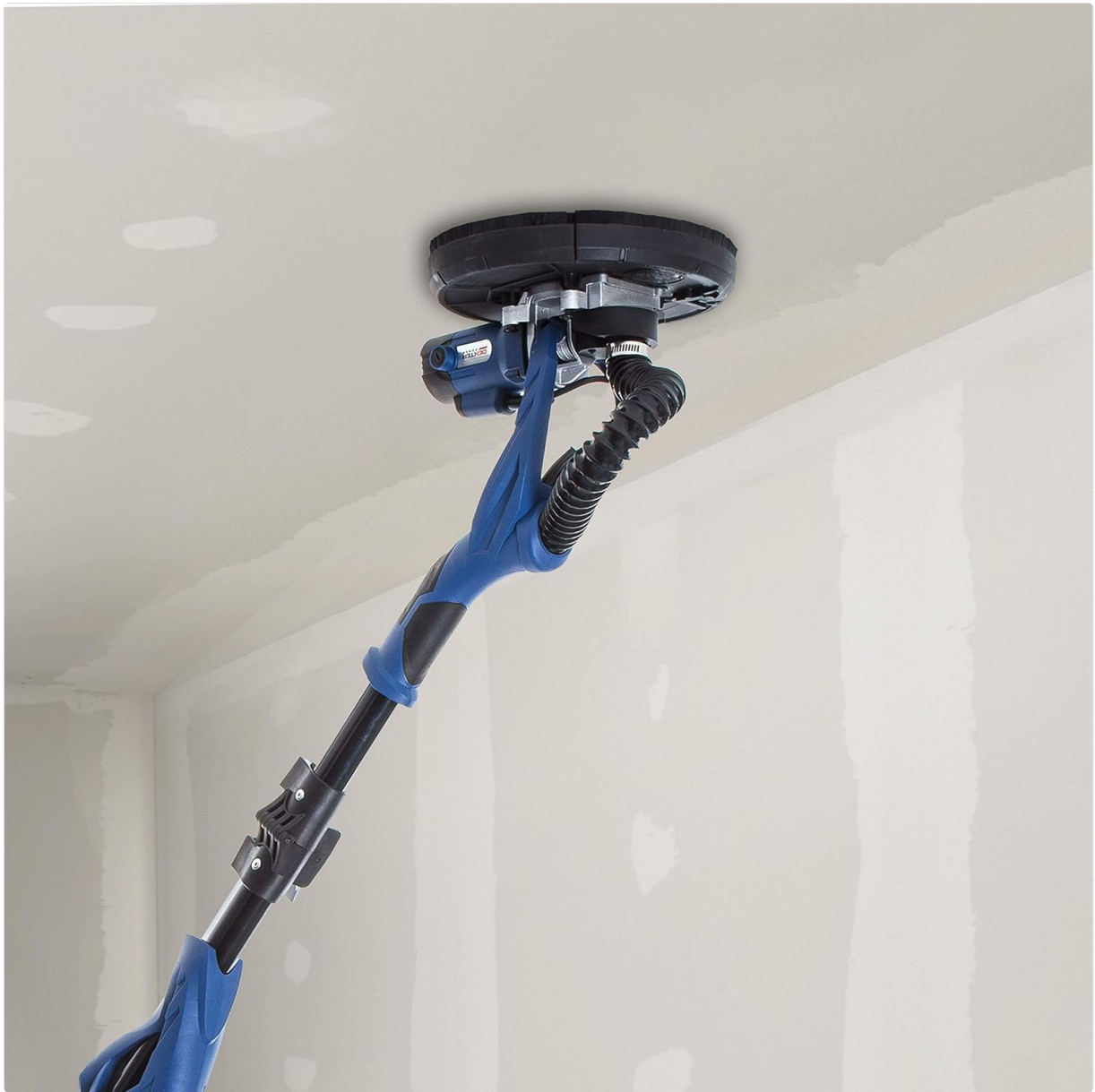
Figure 5: Sander being used to smooth a wall surface.
