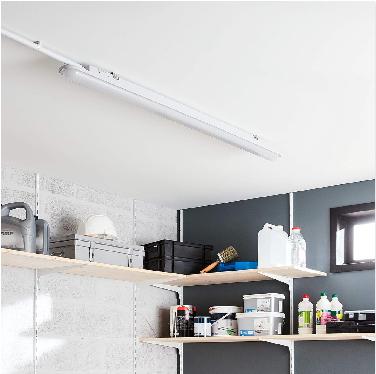
Figure 6: INSPIRE VOLGA LED Lamp installed in a garage, powered off.
