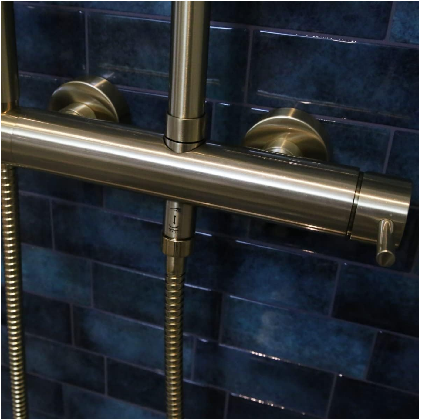
Figure 4: The diverter knob allows switching between the overhead shower and hand shower.
