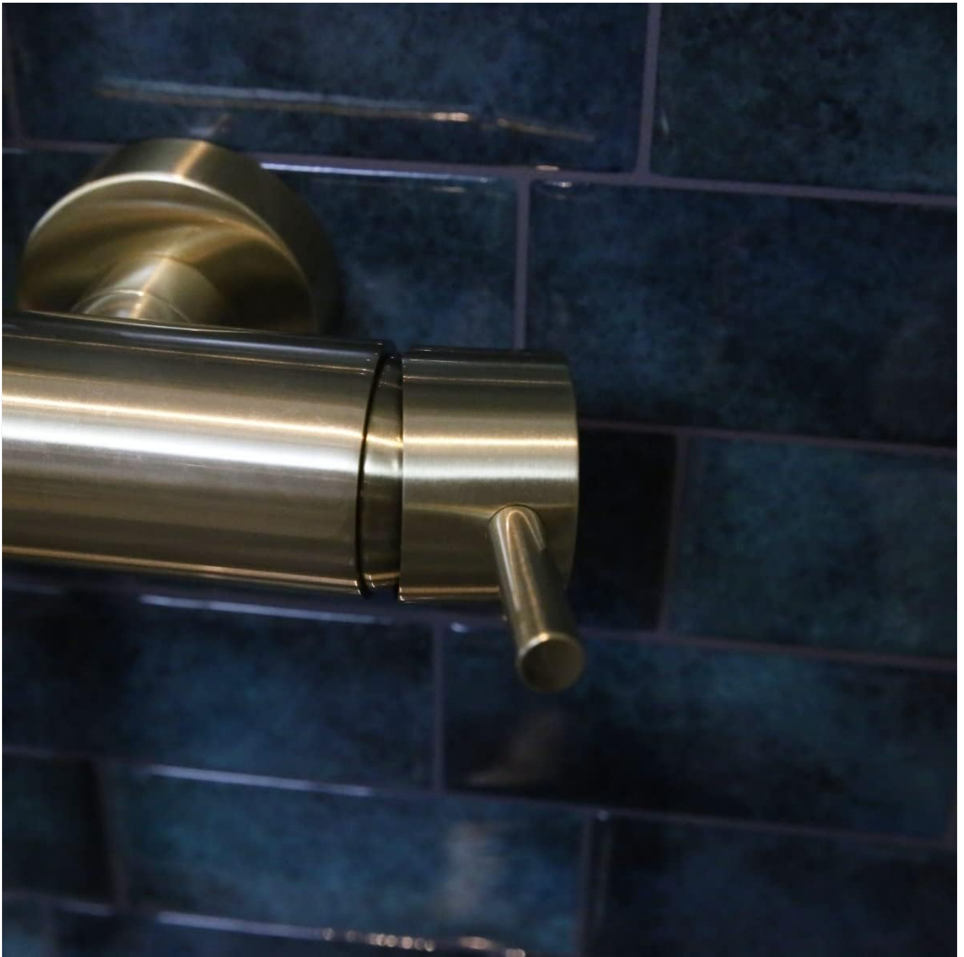
Figure 3: Close-up view of the mechanical mixer handle for temperature and flow control.
