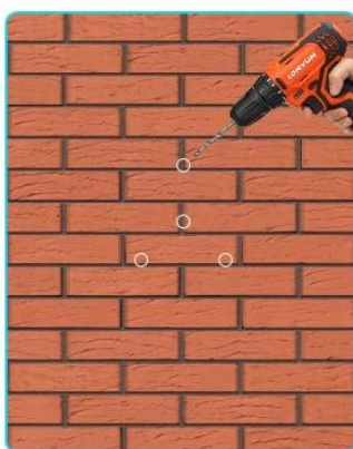
2. Drilling four holes
