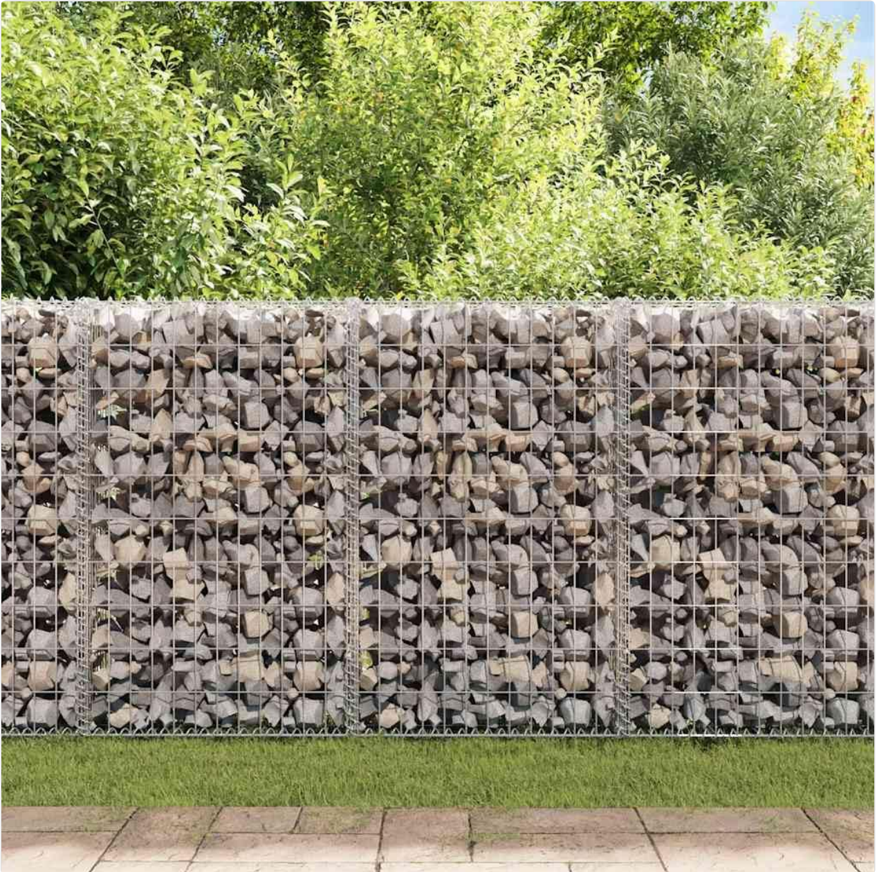
Figure 5.1: A different angle of the gabion wall, showcasing its integration into the natural environment and its robust appearance when filled.
