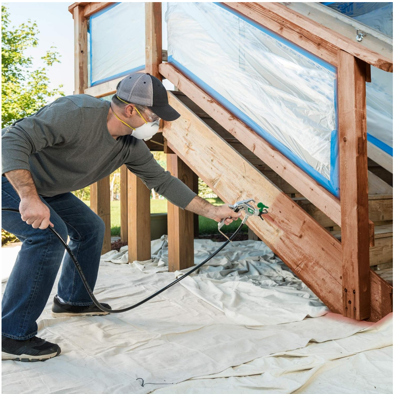
Image 5.3: Applying stain to a wooden deck railing, showing versatility for different materials and applications.
