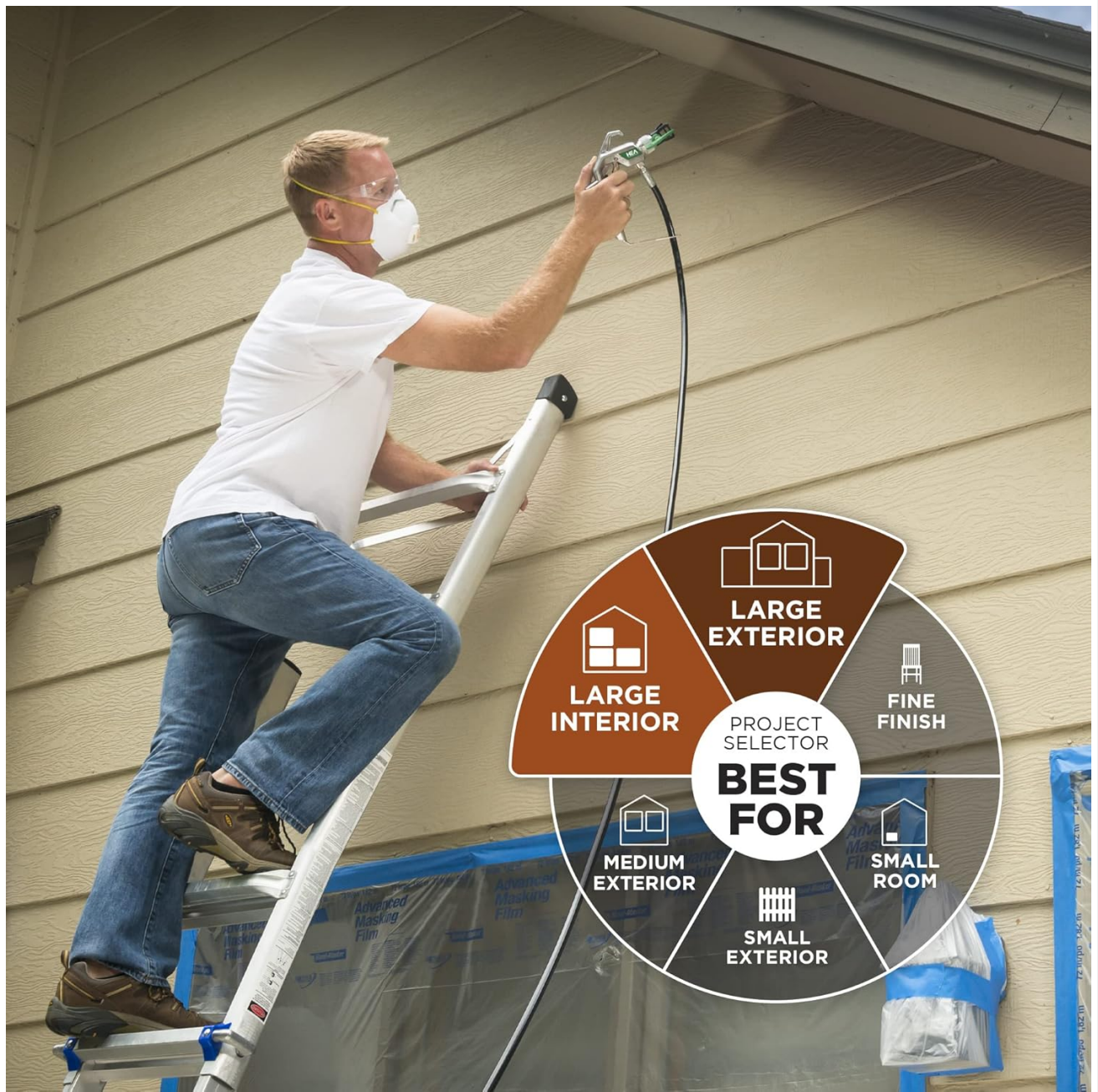
Image 5.1: An operator using the Control Pro 190 to paint exterior siding, demonstrating typical usage for large projects.
