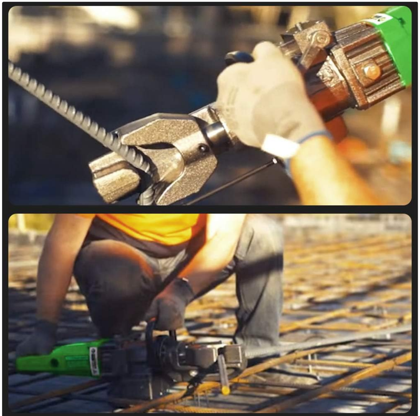
Figure 4.2: The rebar bender in operation, demonstrating how rebar is positioned and bent.
