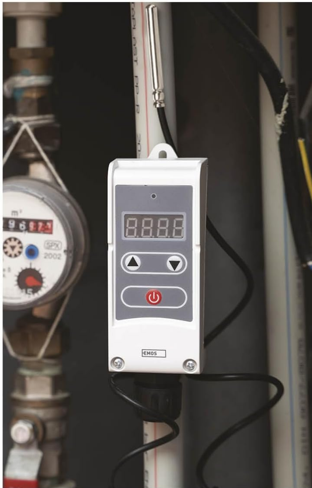
Image 5.1: Example of the EMOS P5684 thermostat installed, showing the unit and remote sensor in a typical application.
