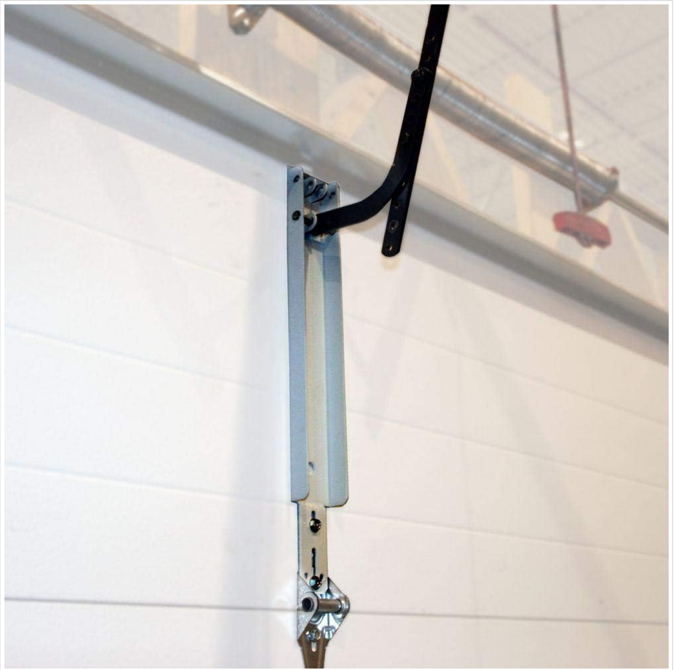
Image: The DURA-LIFT reinforcement bracket, along with the included self-tapping screws, clevis pin, and cotter pin.
