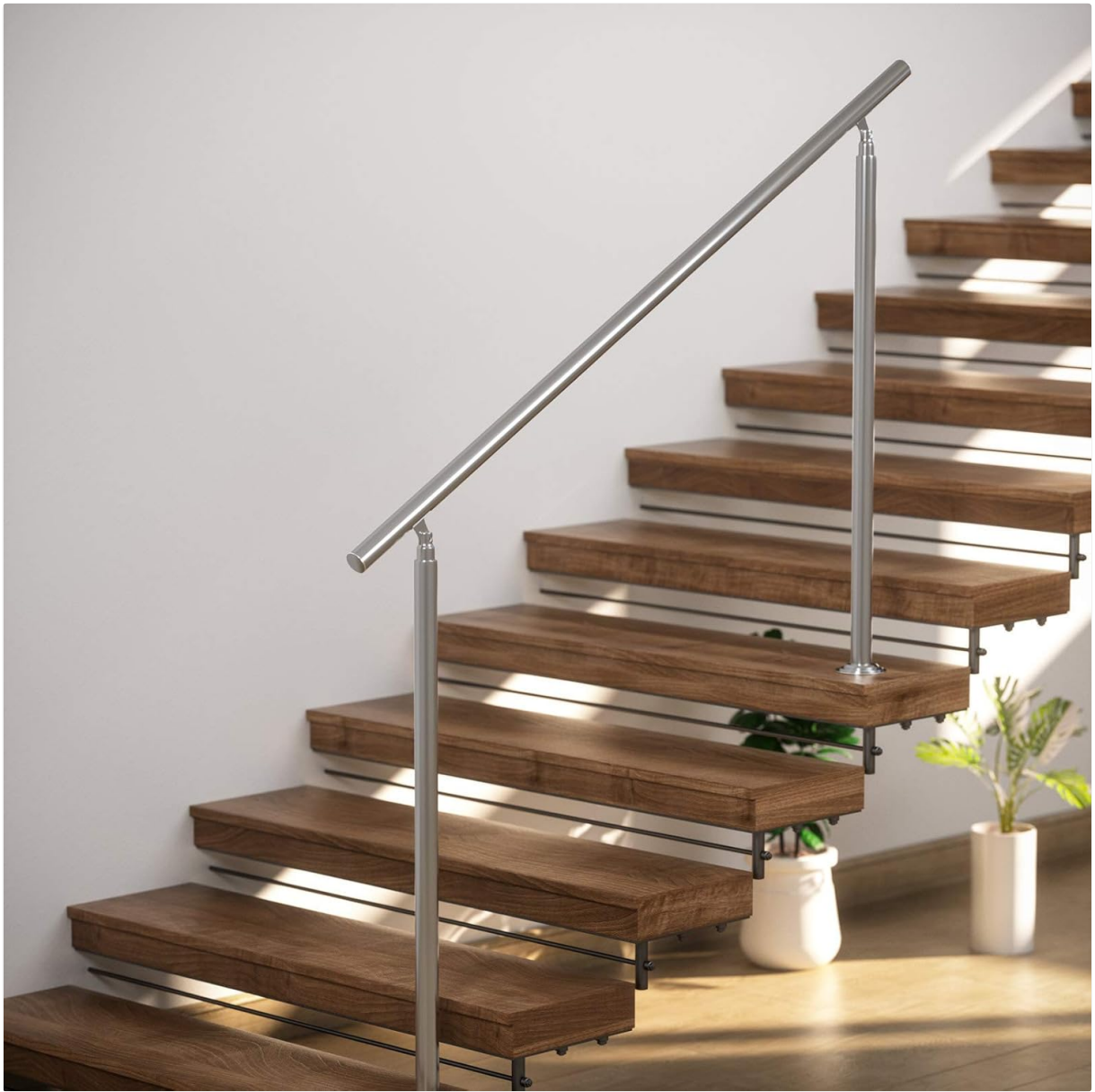
Image 5.2: Handrail providing support on indoor wooden stairs.
