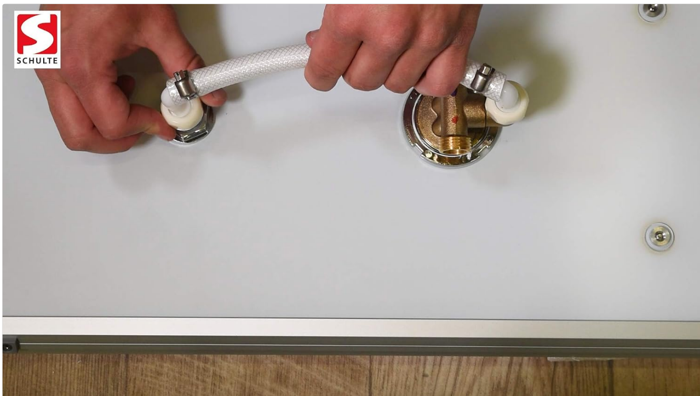
Image: Hands connecting flexible water hoses to the back of the shower column's faucet unit.
