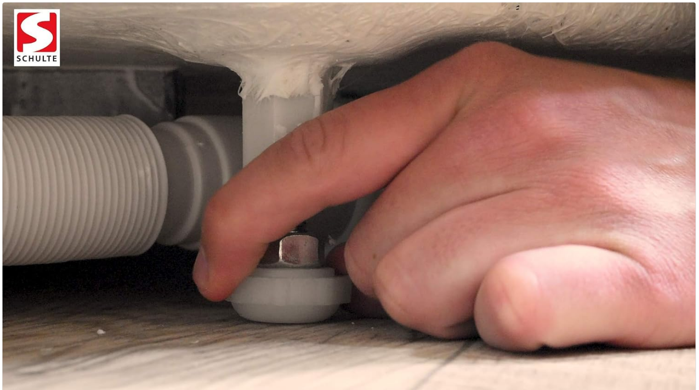
Image: Connecting the shower drain pipe to the shower tray. Ensure all connections are tight and sealed.
