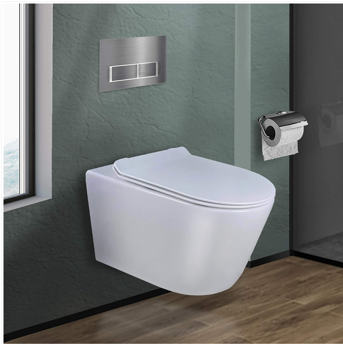
Figure 1: Installed Fine Fixtures Dakota In-Wall Toilet Combo Set.
