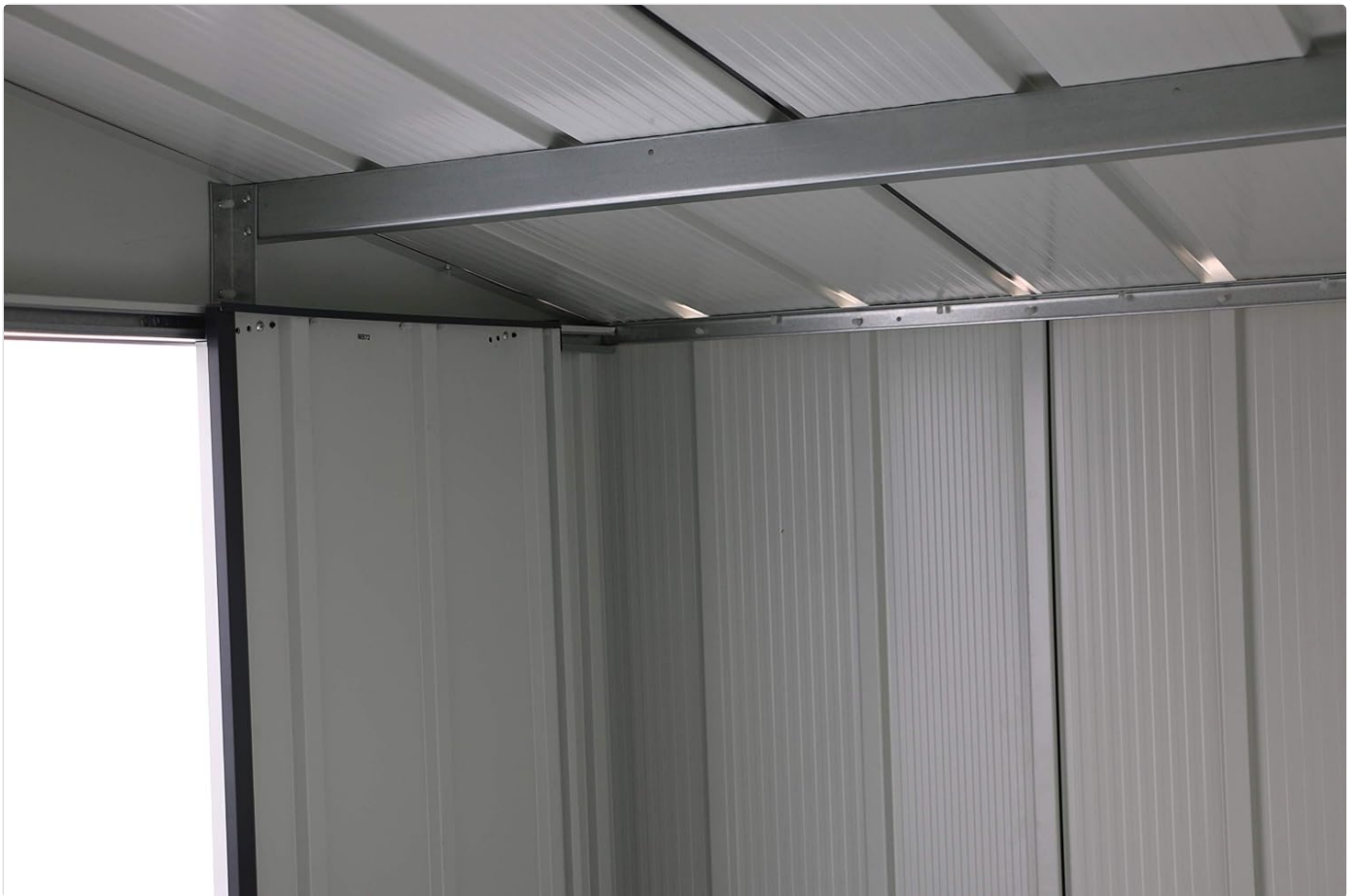
Image 5.1: Interior view of the shed, highlighting the structure of the roof and wall panels during assembly.
