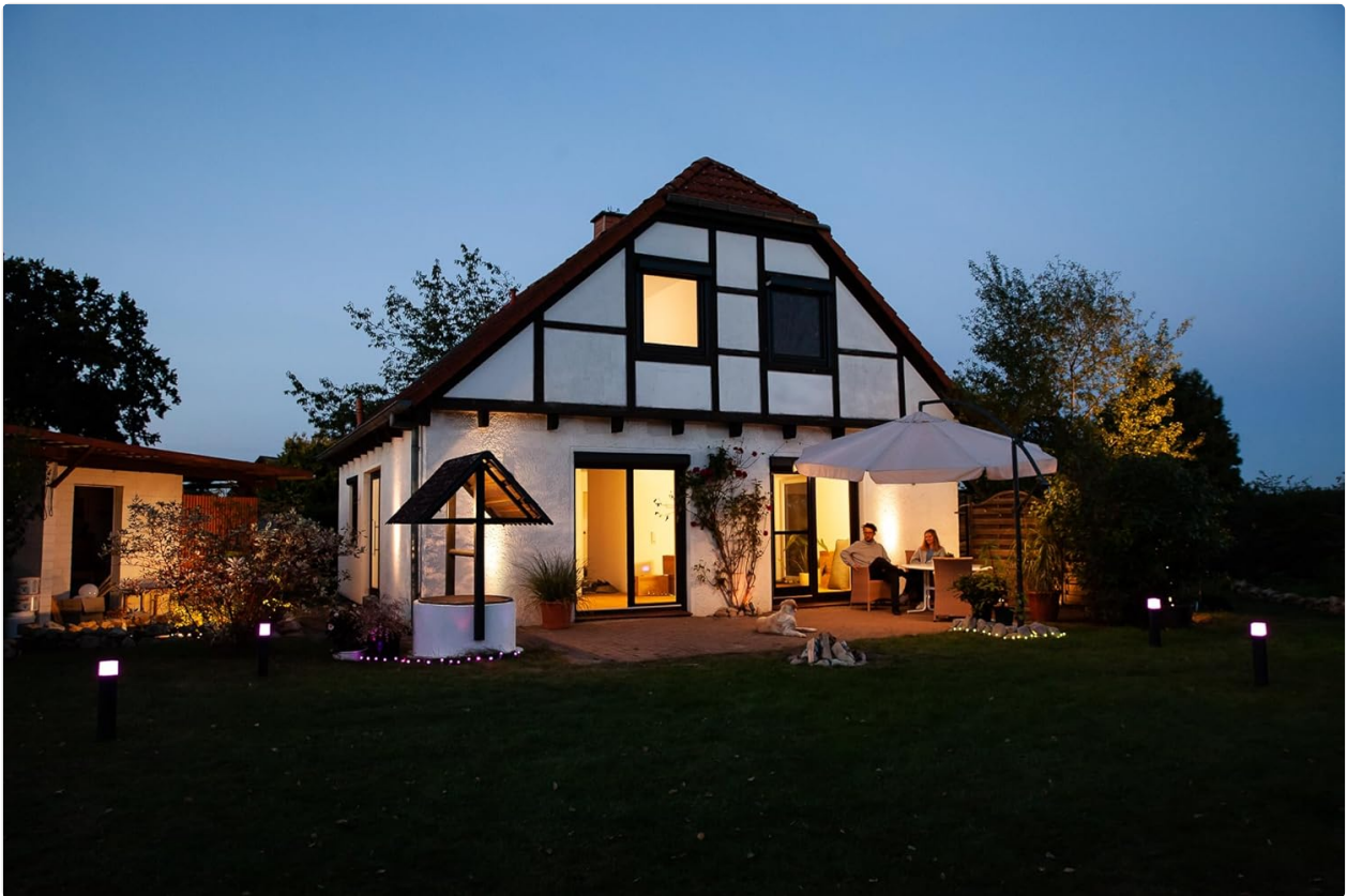
Image 2.1: The LEDVANCE Smart LED Floodlight installed on an exterior wall, providing illumination.
