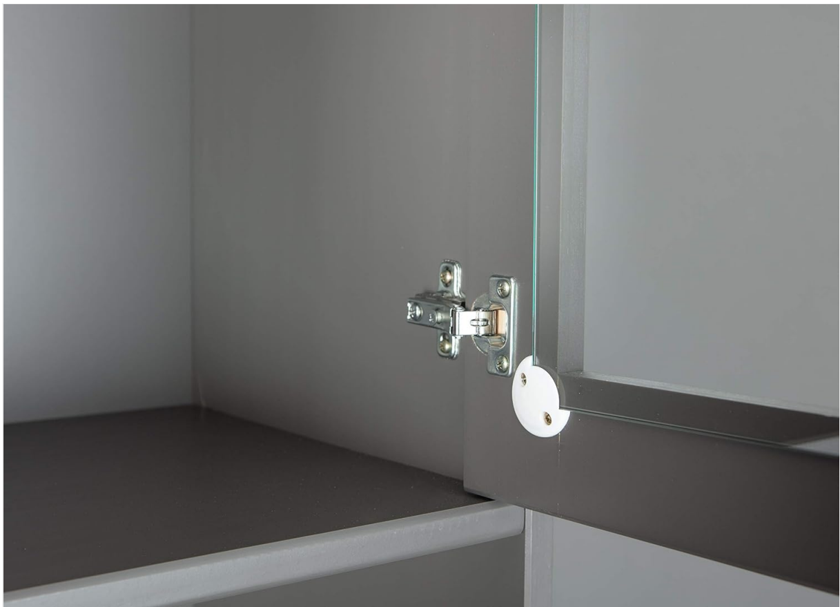
Figure 2.4: Detail of a cabinet door hinge, crucial for proper door function and alignment. Ensure these are installed correctly and tightened.
