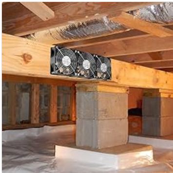
Crawl space ventilation.
