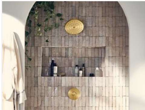
Figure 2: M-CORE valve body secured to a wooden brace within a wall opening, ready for plumbing connections.
