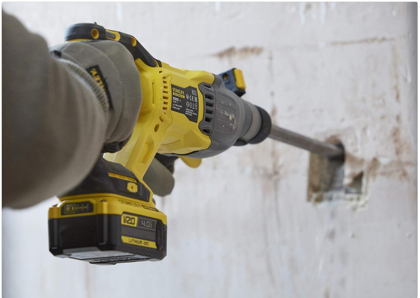
Figure 9: Demonstrating hammer drilling into a wall.
