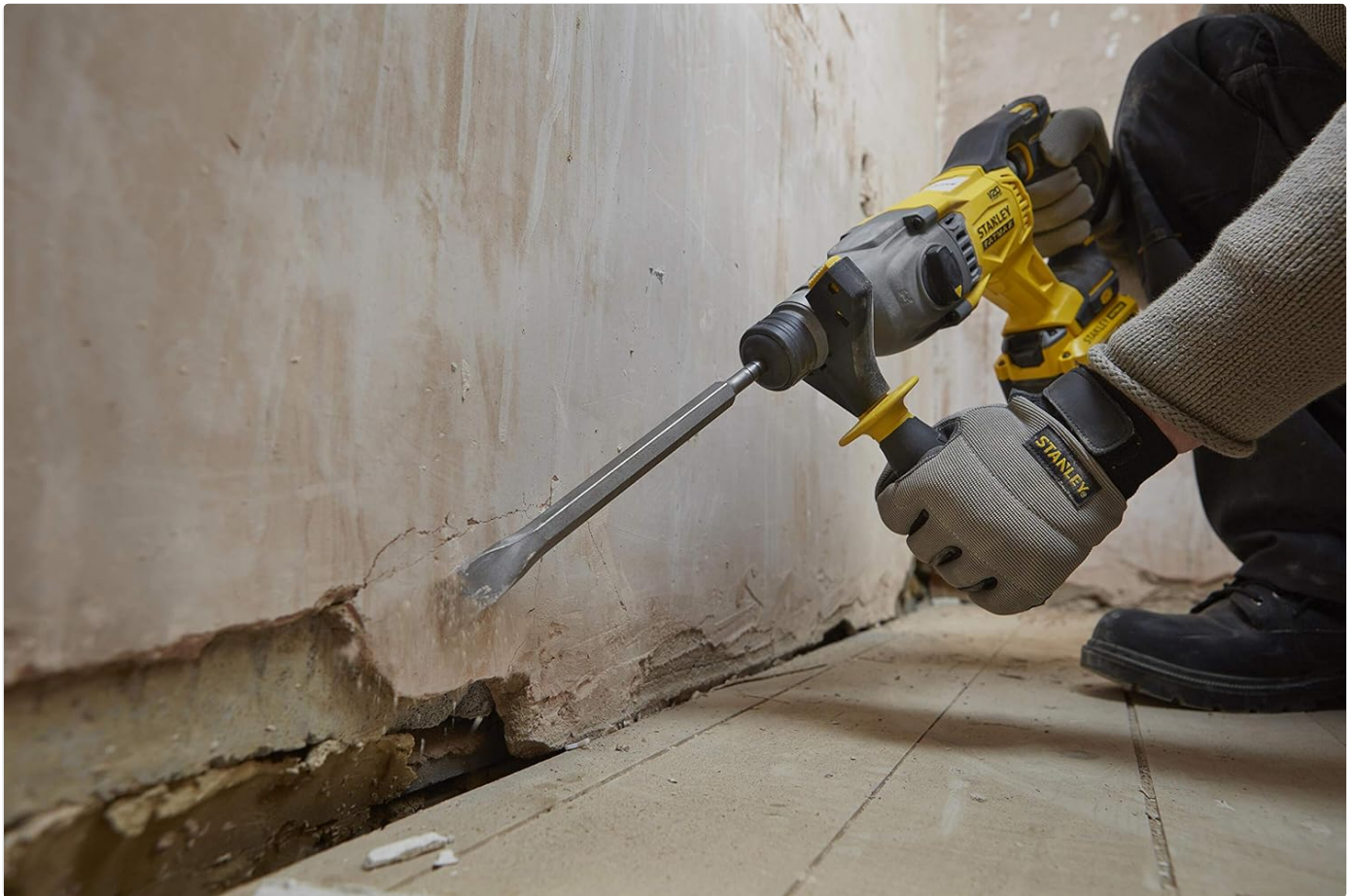
Figure 10: Performing light chiseling work with the tool.
