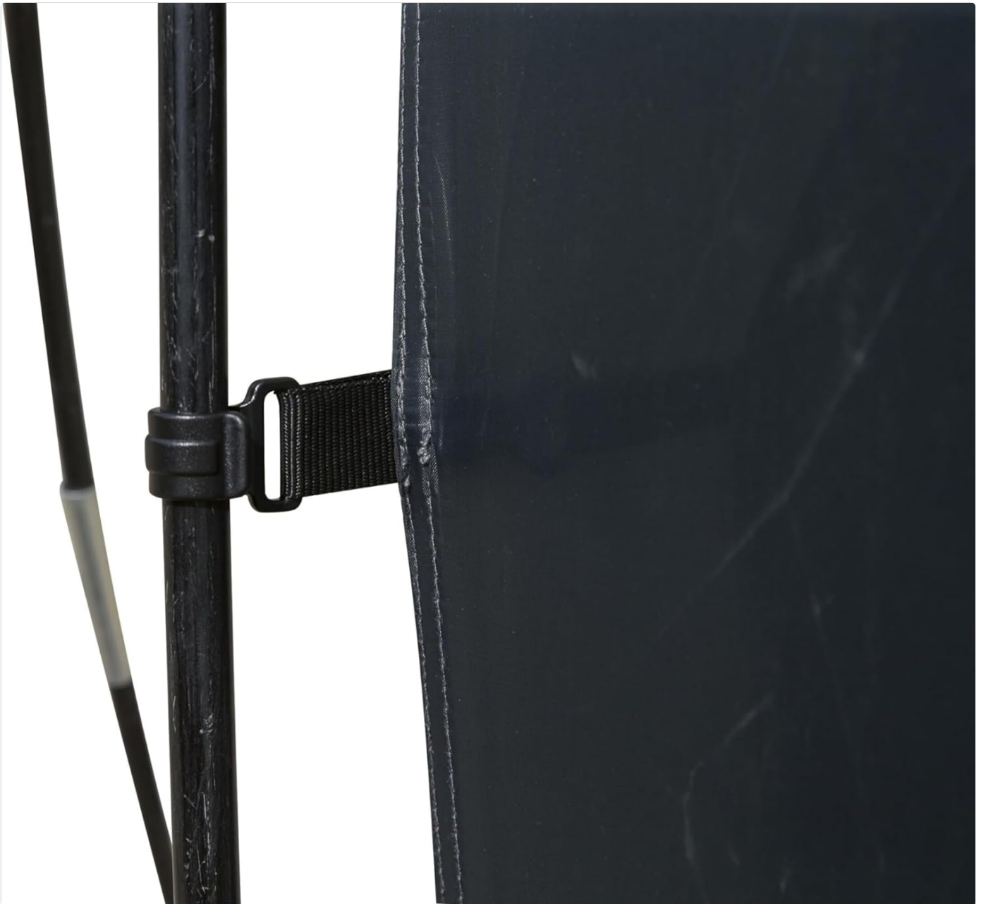
Figure 4.6.1: A close-up of a D-ring attachment point on the interior of the dome, likely used for hanging items or securing internal features.
