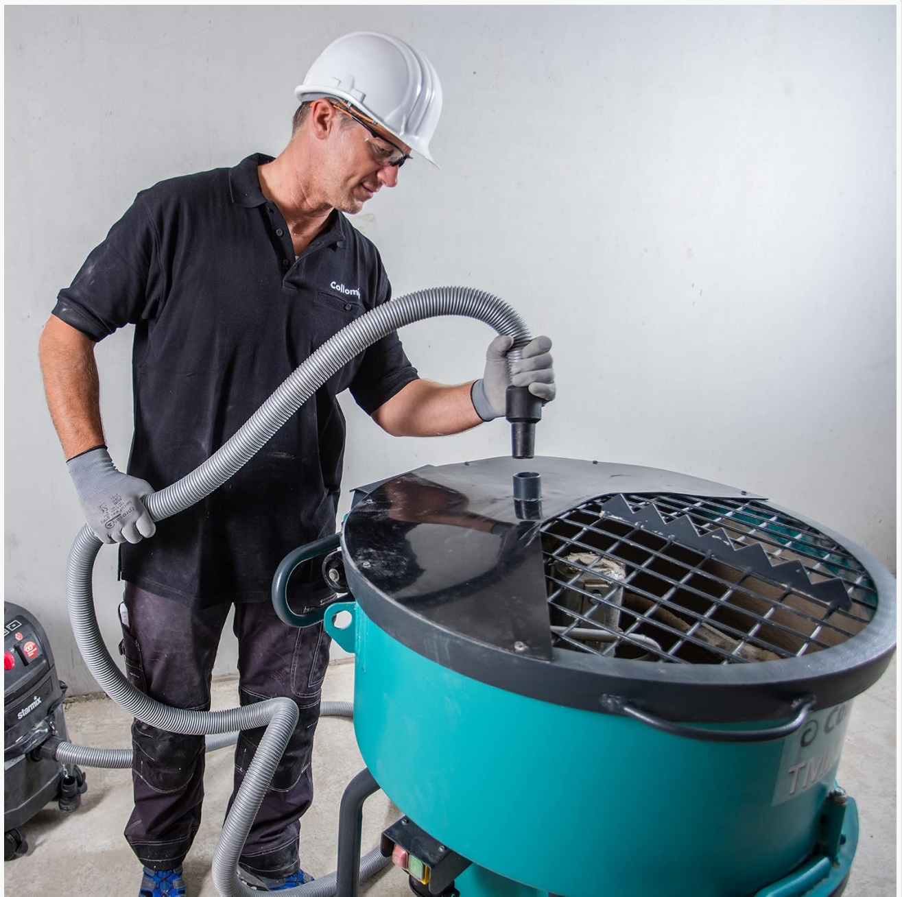
Figure 6: A worker connecting a vacuum hose to the dust extraction port on the TMX1000 mixer to minimize airborne dust.
