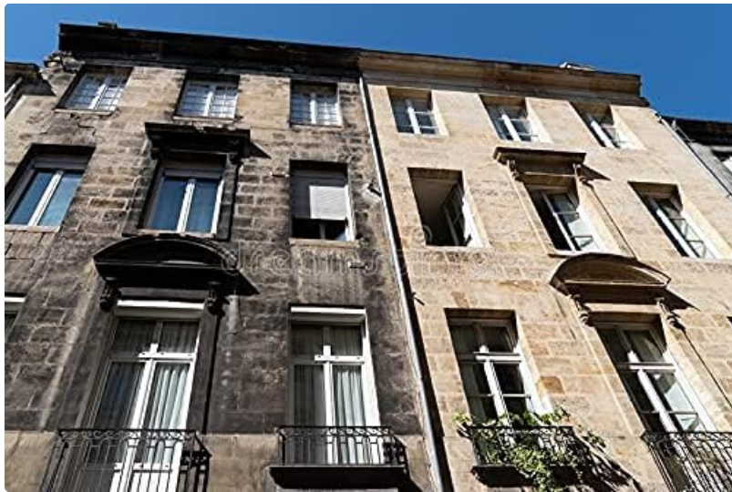
Image: A building facade showing a clear before-and-after comparison of pressure washing, with one side clean and the other still dirty.
