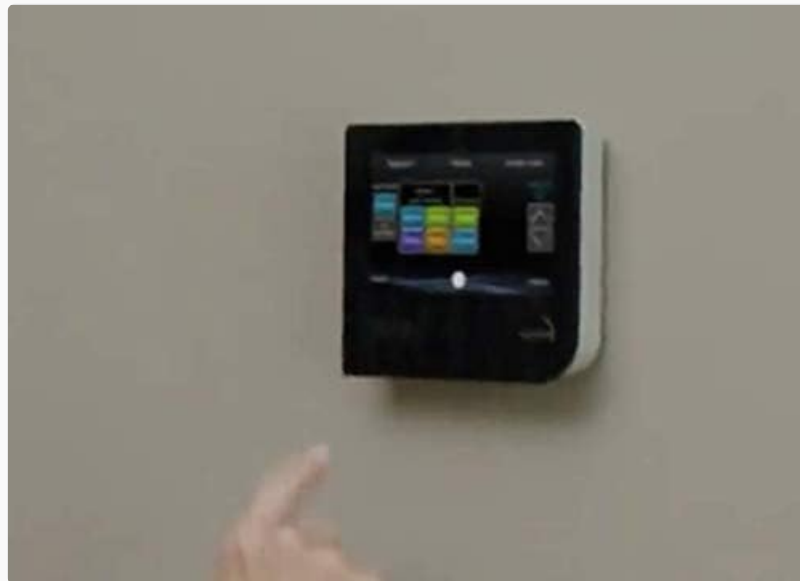
Figure 2: The Carrier Infinity SYSTXCCITC01-B Thermostat installed on a wall, ready for operation.
