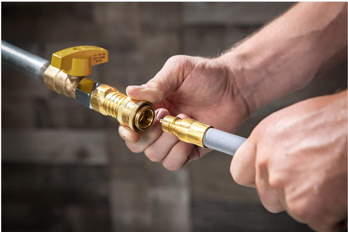
Image 5.3: Demonstrates the process of connecting the quick connect fitting to the natural gas supply line.
