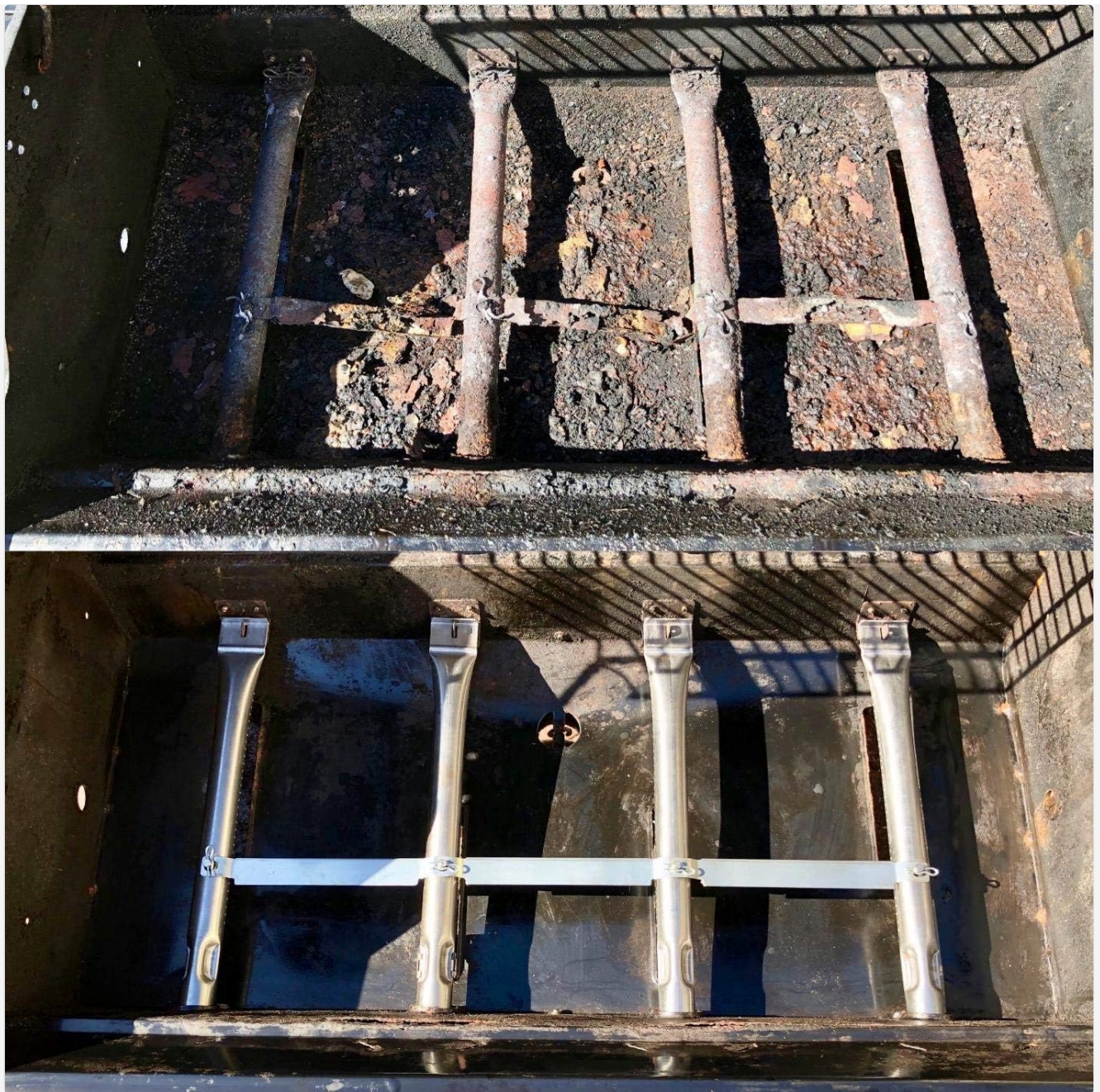
Image 5.1: Comparison of old (top) and new (bottom) burner pipe installation.
