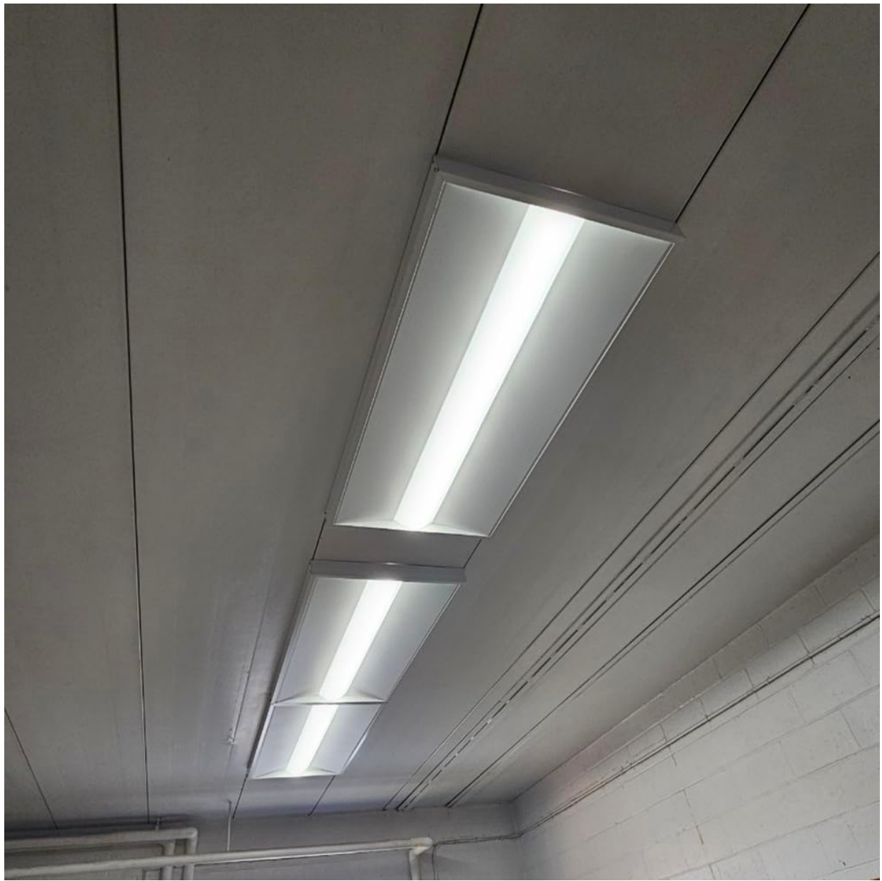
Image 3.3: Example of installed LED panels using the surface mount frame kits.
