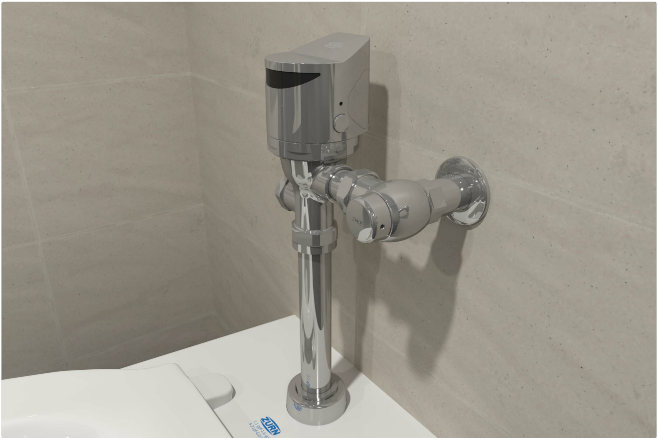
Figure 7: Close-up of Installed Flush Valve
