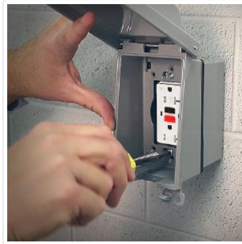
Image: An example of installing the GFCI outlet into a weatherproof outdoor electrical box.
