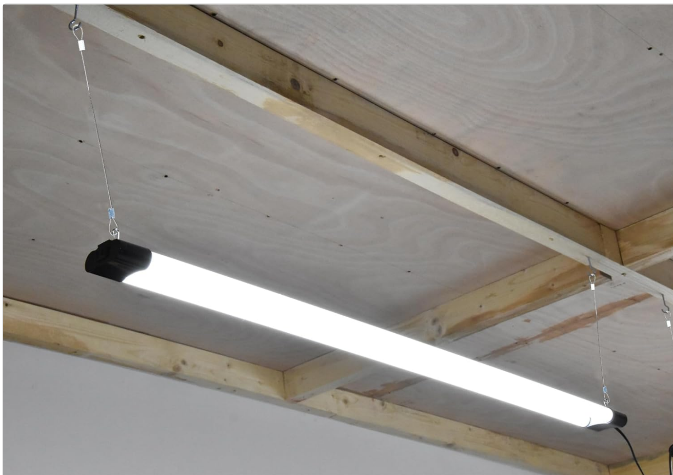
Image: Example of a hanging mount installation in a shed.
