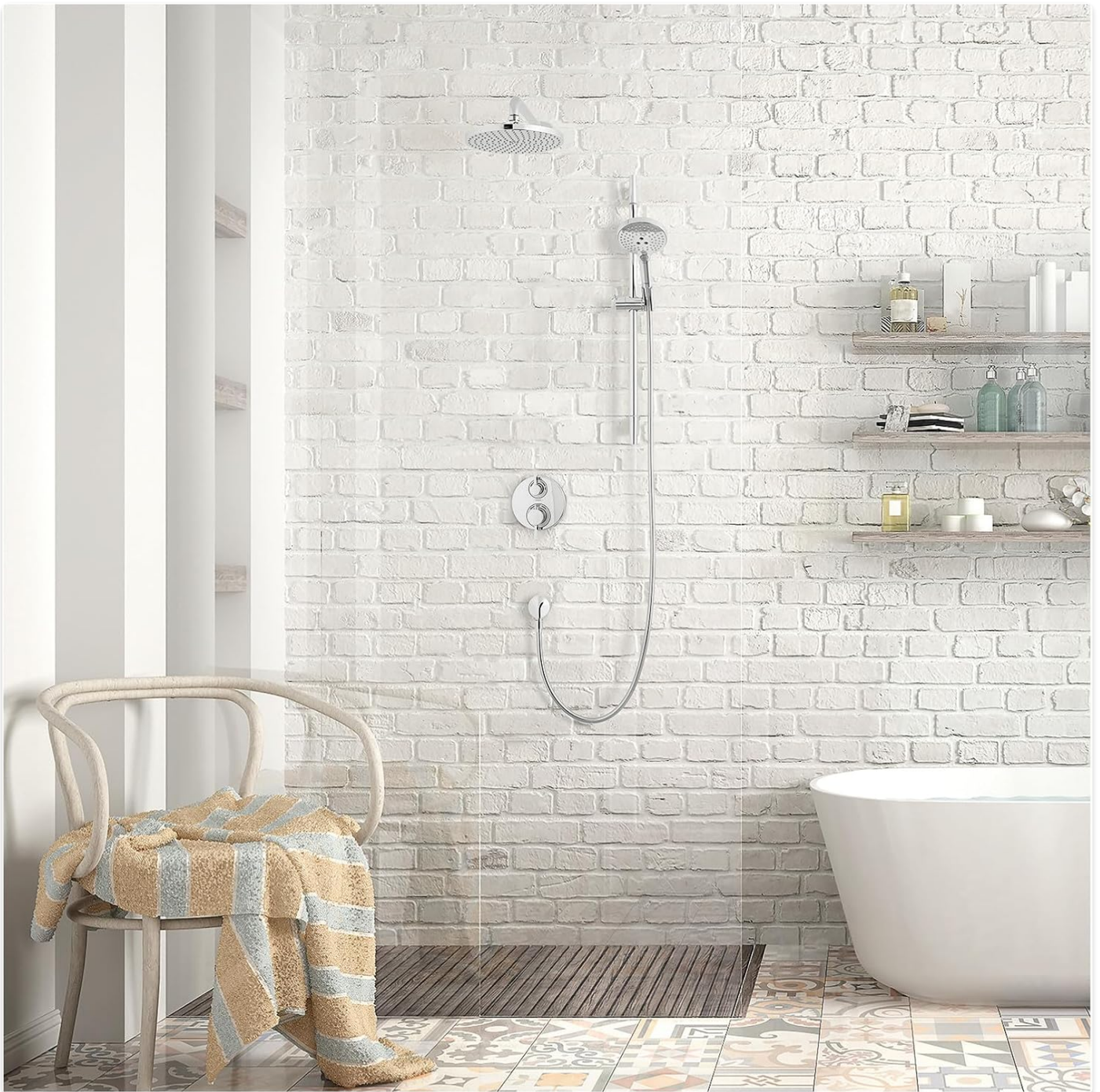
Figure 1: The hansgrohe Raindance S Complete Shower System installed in a modern bathroom setting.
