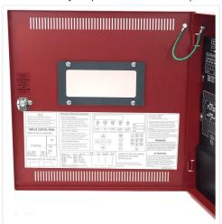
The inside of the panel door provides a quick reference guide for emergency operation procedures and a layout of the control buttons. This includes instructions on how to acknowledge alarms, silence signals, and reset the system.
