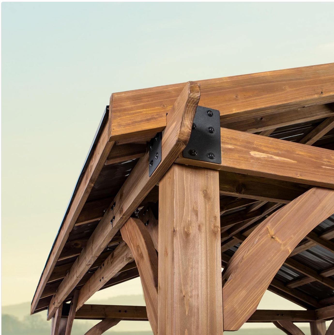
Image: A detailed view of the gazebo's wooden frame and the connection points to the steel roof, highlighting the craftsmanship and robust construction.
