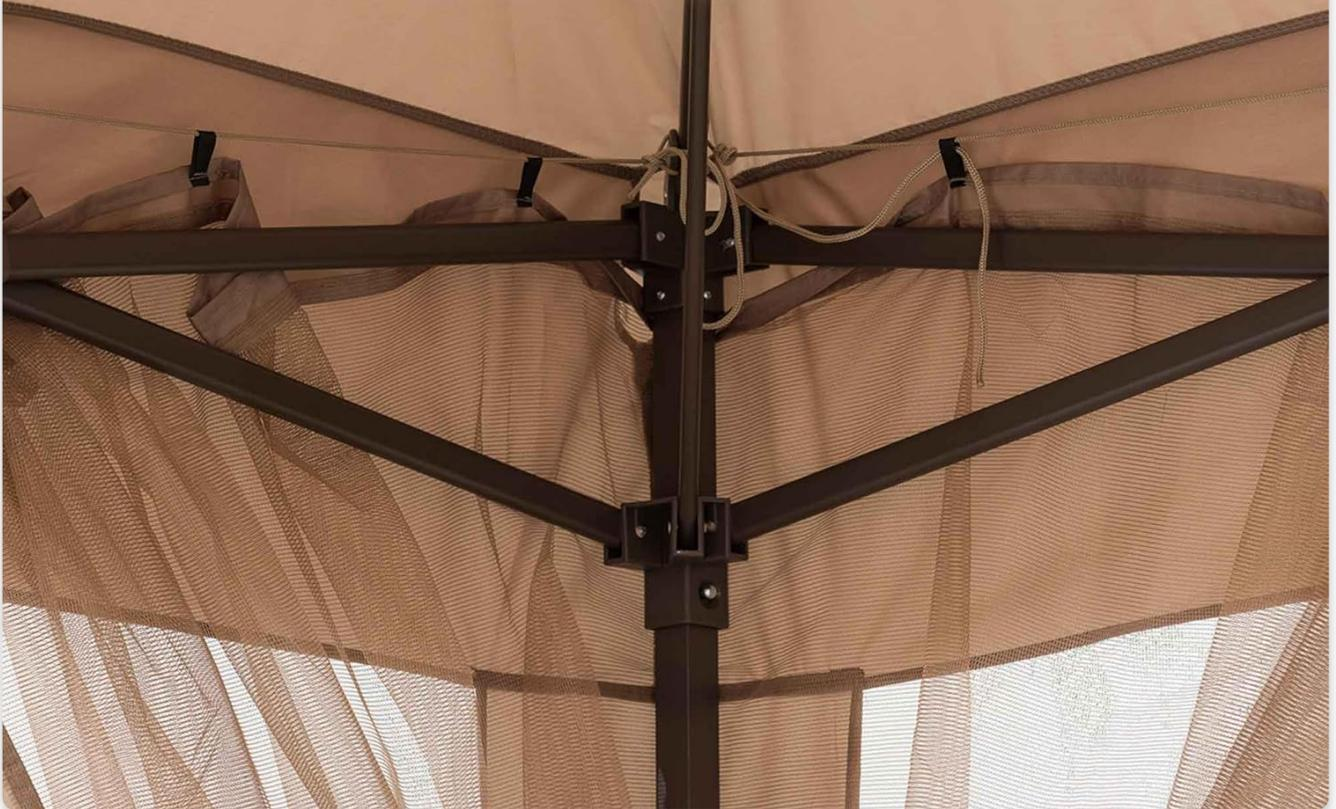
*Figure 3: Detail of the powder-coated steel frame structure.*
